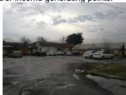
Proposed location for the new construction sufficient to accommodate the new building and other secondary structures. Building on the back is existing SESS
