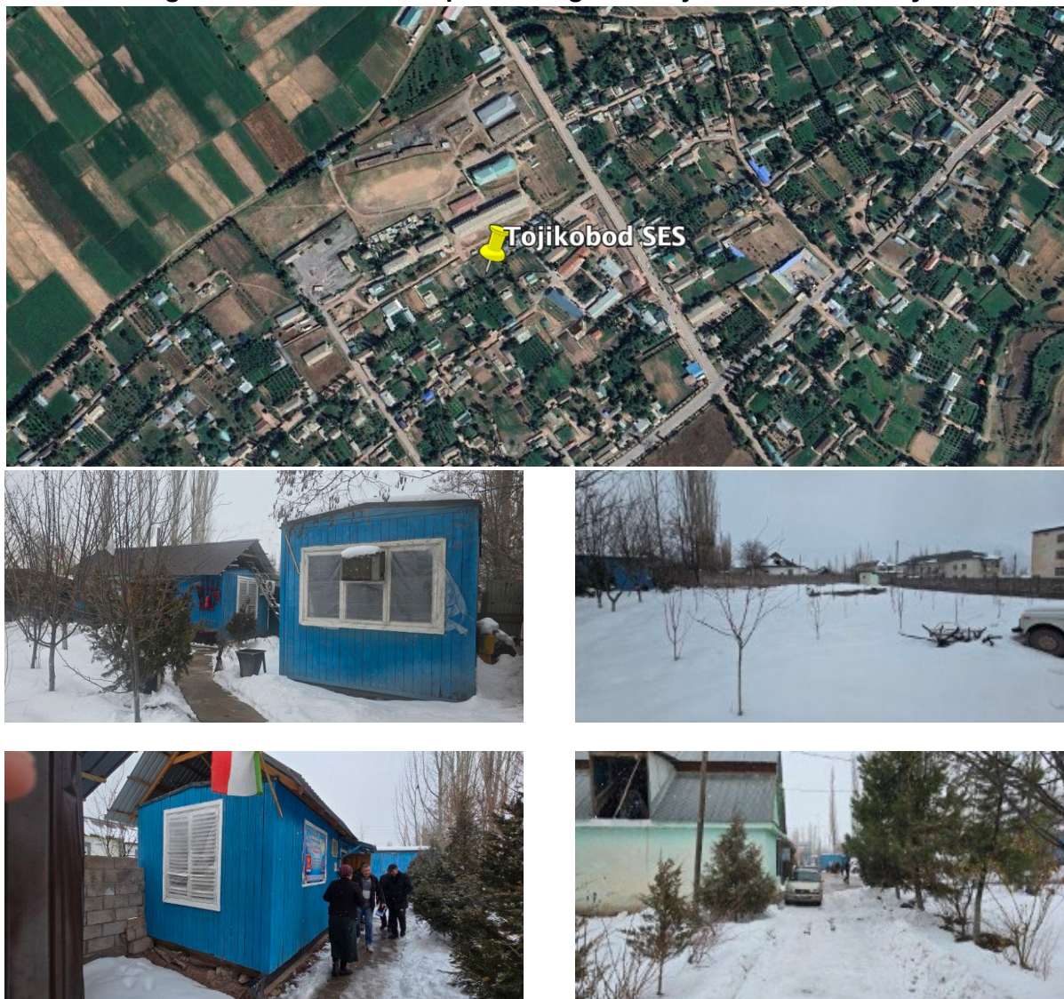
Figure IV-2: Location map and images of Tojikobod SES facility
