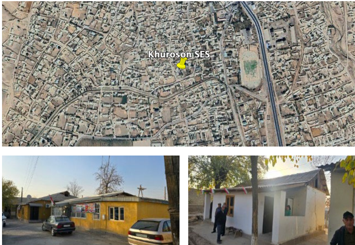
Figure IV-9: Location map and images of Khuroson SES facility
