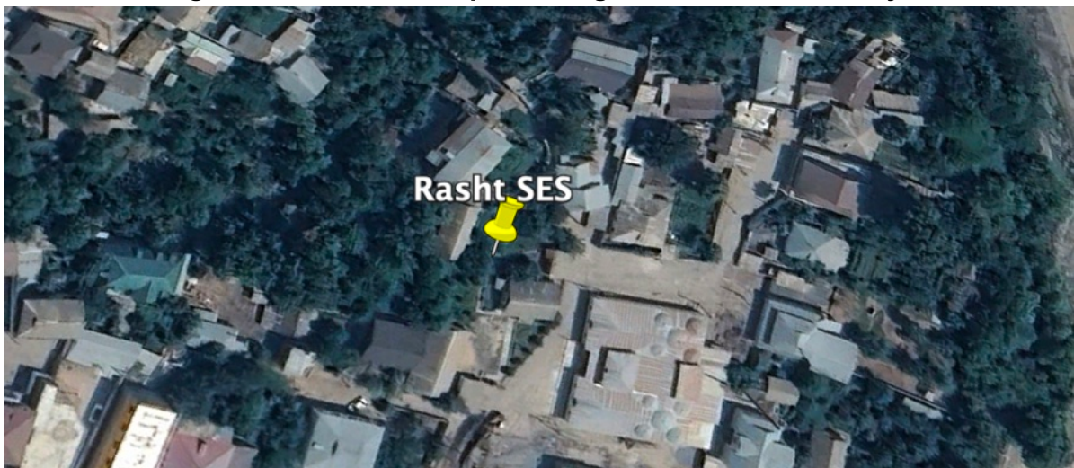
Figure III-1: Location map and images of Rasht SES facility
