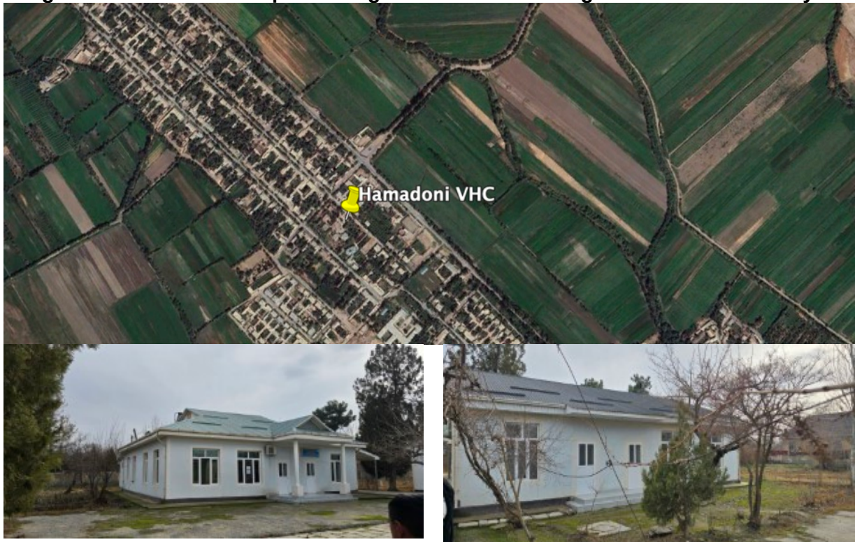
Figure III-10: Location map and images of Hamadoni Village Health Center facility
