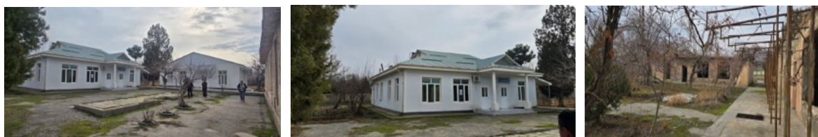
Photos of the Consultation Process in Bahoriston village Rural Health House location
