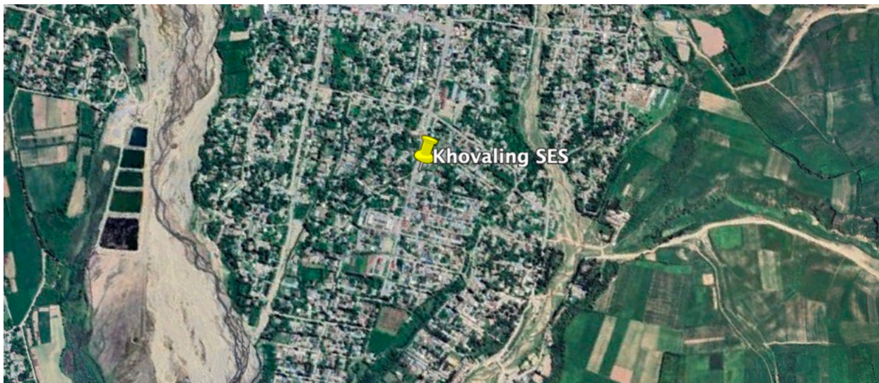
Figure III-5: Location map and images of Khovaling SES facility
